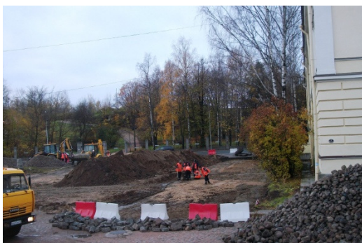
October 2010, Workmen begin rebuilding the square in front of our Christian Center
