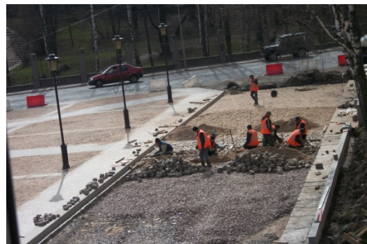
May 2011, laying old cobblestones in the new street (17 th Century technology) Judy has been witnessing to the workmen with cakes, clothes, and Christian literature.
